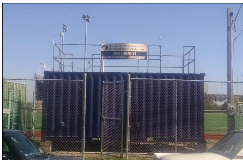
Figure 2-1 Bayonne Air Monitoring Station
